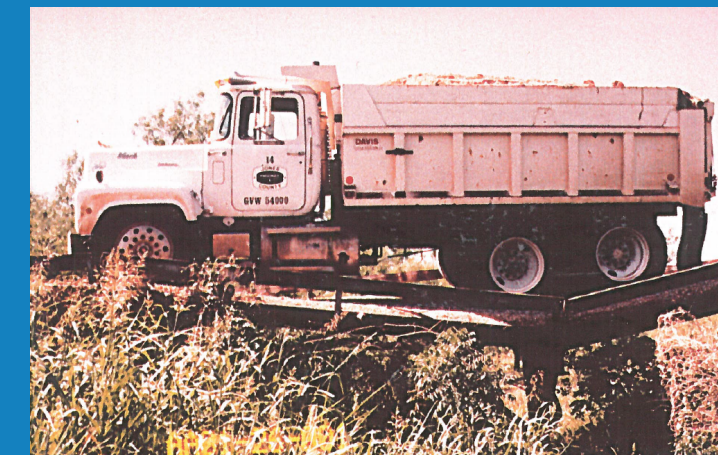
Photo 1 – The capacity of a bridge posted for 12,500 lbs was exceeded under loading from a truck with gross vehicle weight of 54,000 lbs in 1996.
